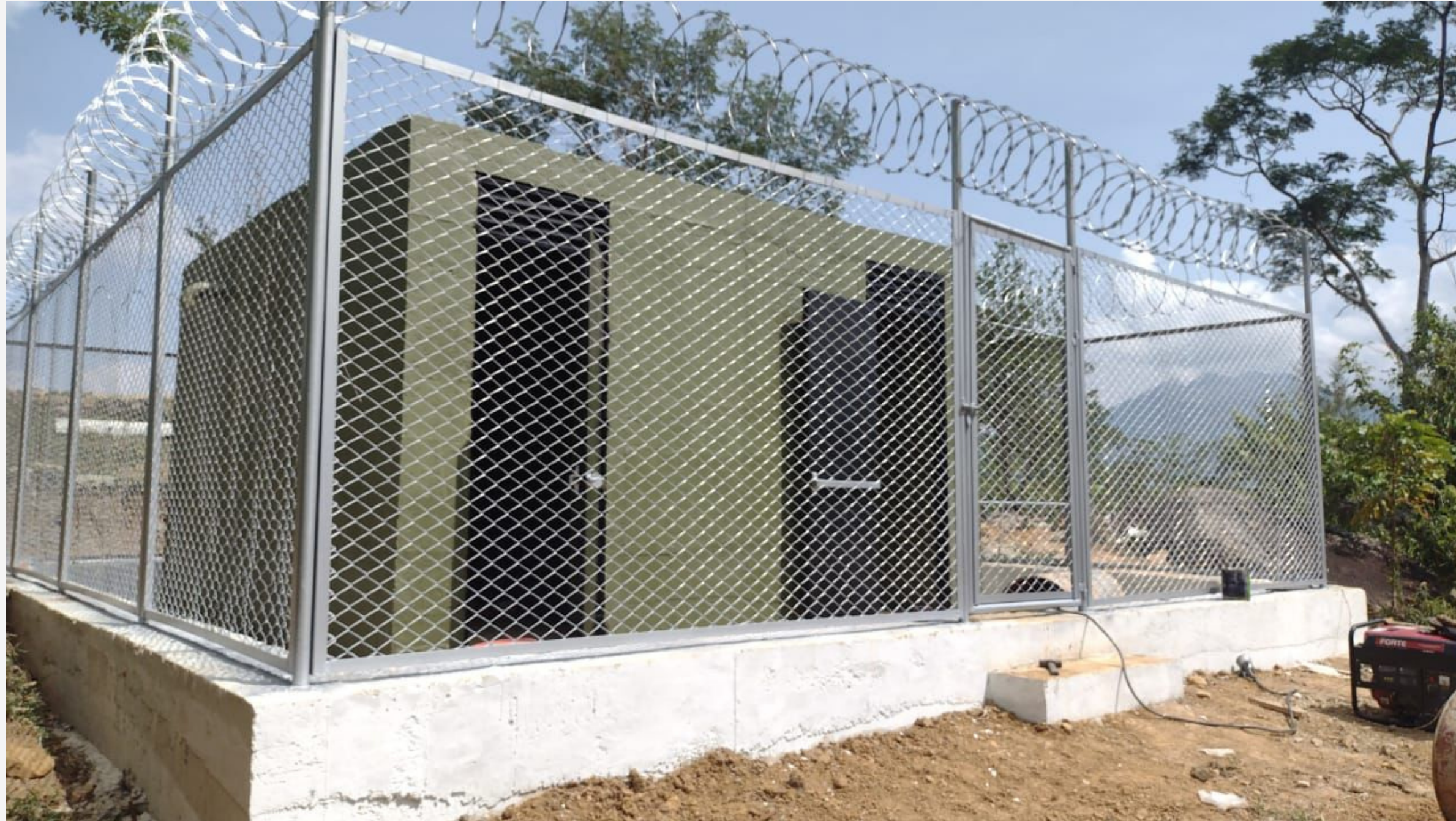
Completed - construction of the powder magazine
