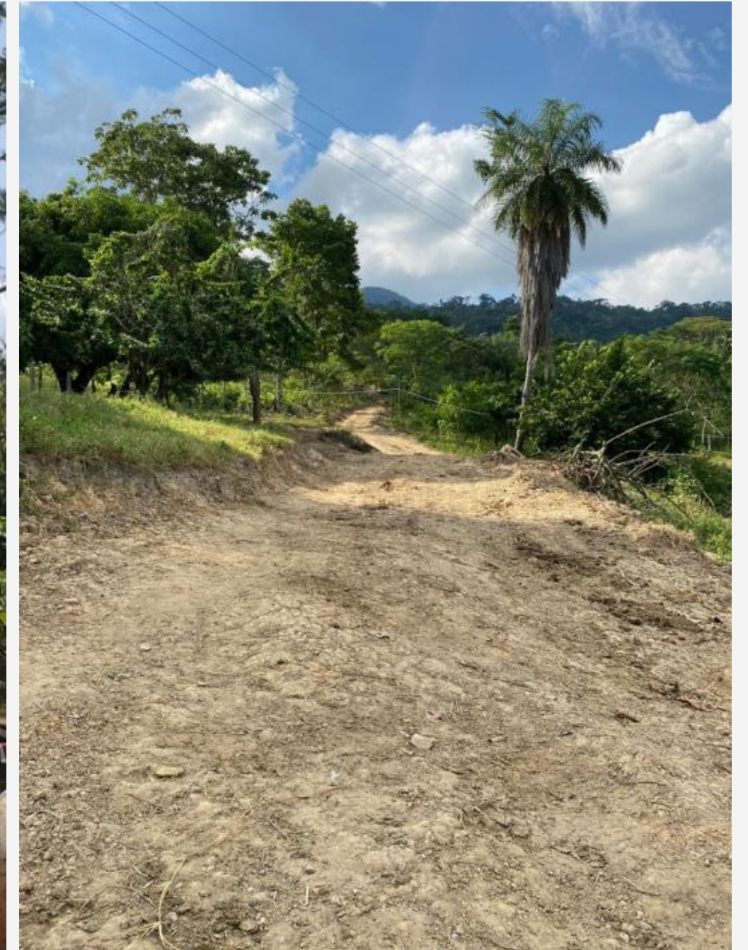
Ongoing – Road construction
