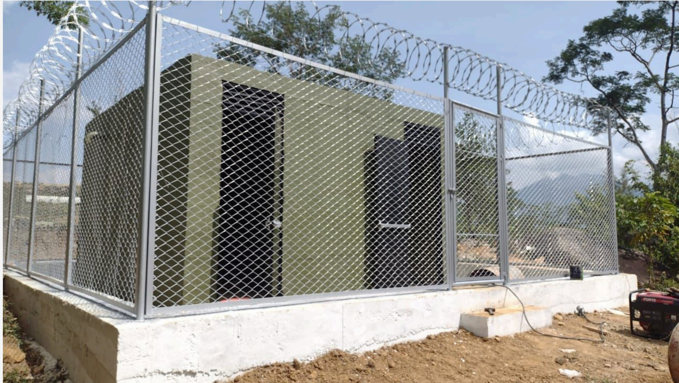
Completed - construction of the powder magazine
